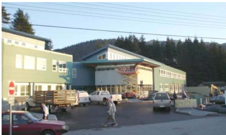
Exterior of South Building
